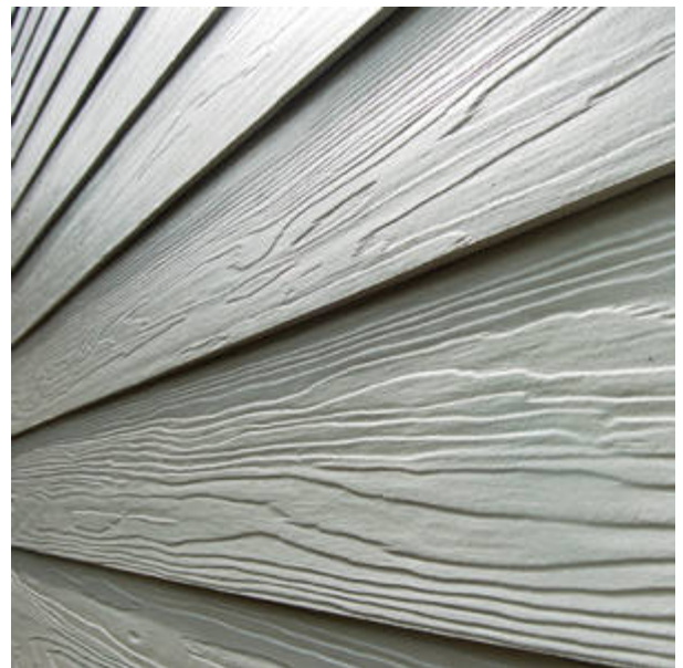
Fiber cement (also called "Hardy Plank") is an approved siding material in certain cases.
