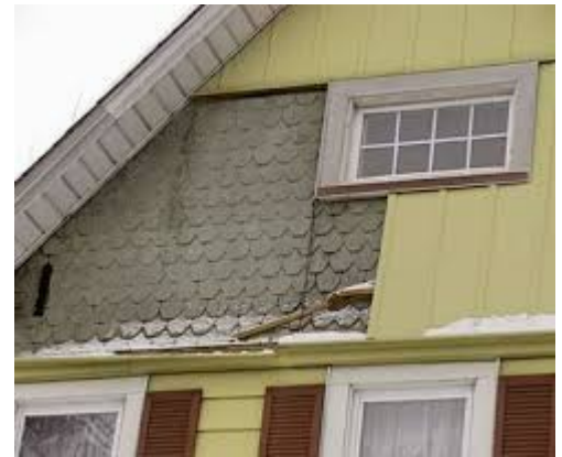
Covering the original materials often conceals the original design intent and workmanship associated with the house.
